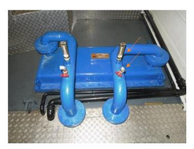
pressure (depression) at the suction side of the cooling water pump and that the pressure difference over the box-cooler was significantly higher than what the box-cooler manufacturer allows.
